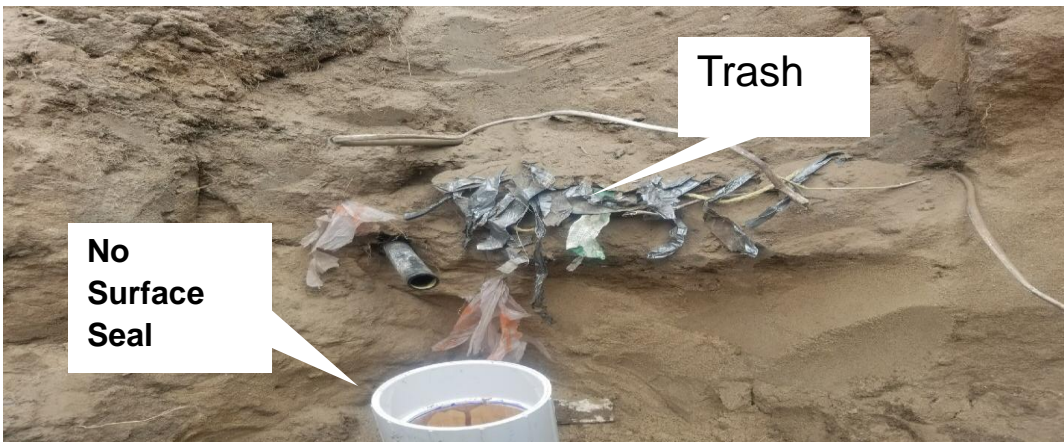
These photos show poor quality of workmanship which can allow potential contamination of ground water.
