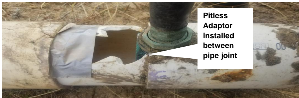
These photos show poor quality of workmanship which can allow potential contamination of ground water.
